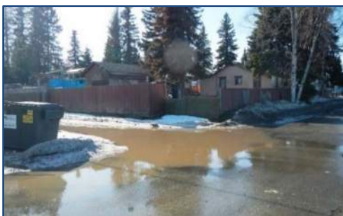
Ponding along W. 32nd Avenue
