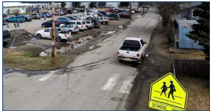
School crosswalk does not connect any pedestrian facilities.
