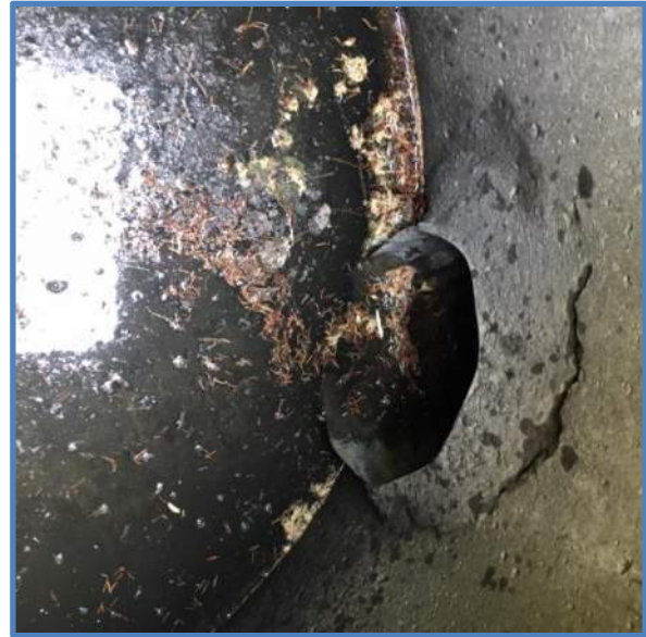
Photo 4 - Outlet Pipe Penetration
