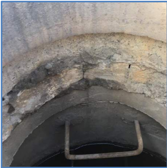
Photo 3 – Frame, Brick Grade Ring, Reducing Slab, and Ladder Rung
