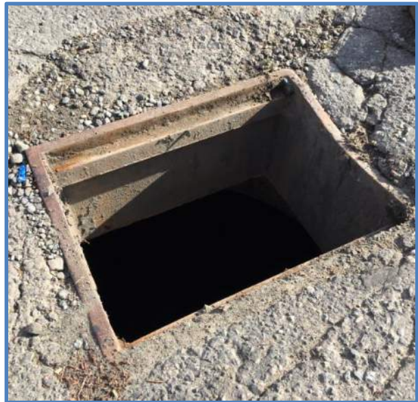
Photo 4 - Frame & Reducing Slab
