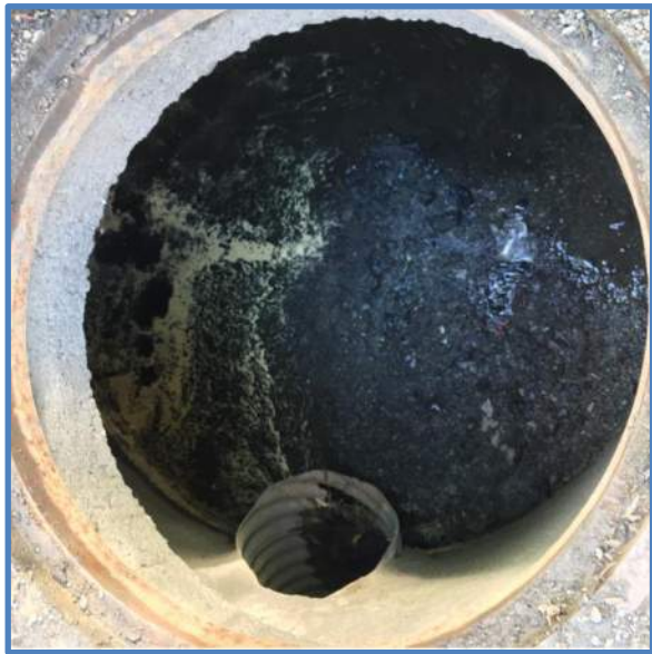
Photo 3 - Frame, Reducing Slab & Outlet Pipe
