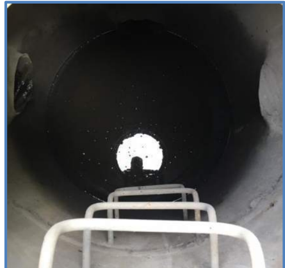
Photo 5 - Inlet & Outlet Pipe Penetrations & Ladder Rungs
