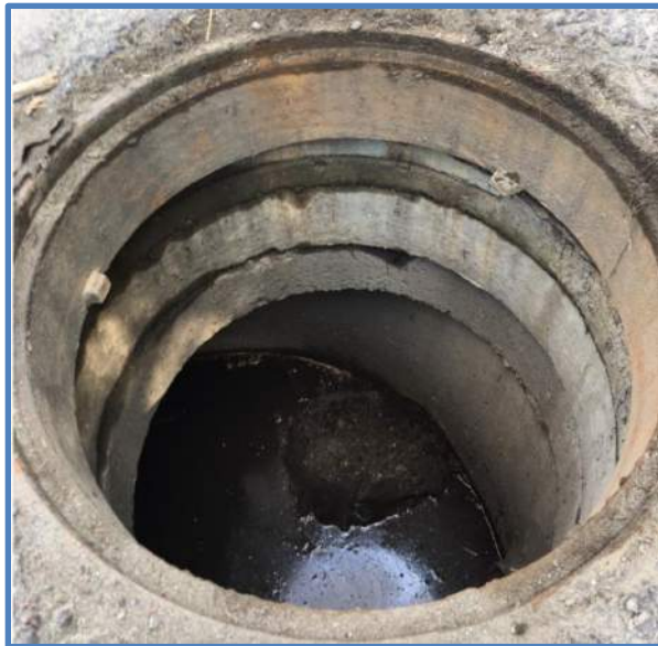
Photo 3 - Frame, Grade Rings & Reducing Slab
