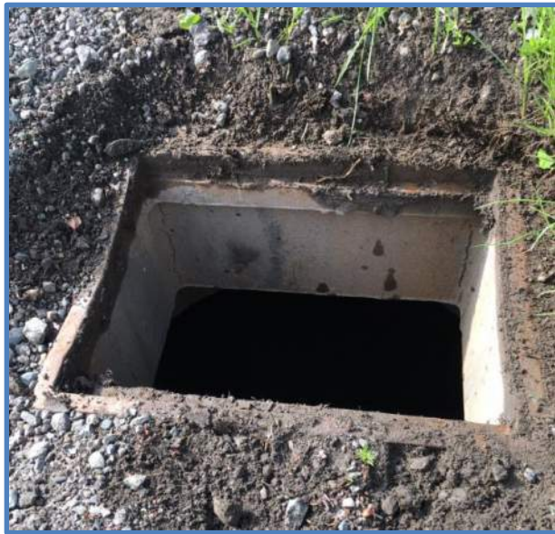
Photo 3 - Frame & Reducing Slab
