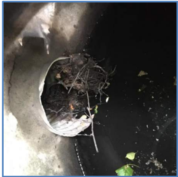
Photo 4 - Outlet Pipe Penetration
