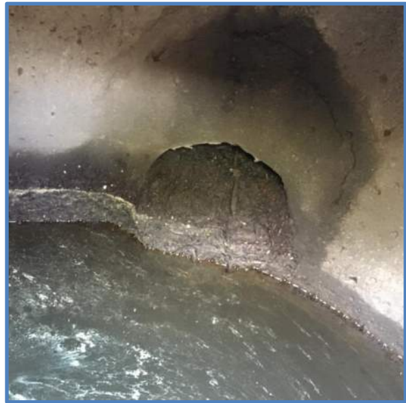
Photo 4 - Inlet Pipe & Pipe Penetration
