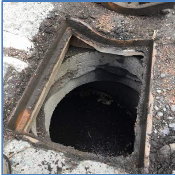
Photo 3 - Frame, Grade Rings & Reducing Slab
