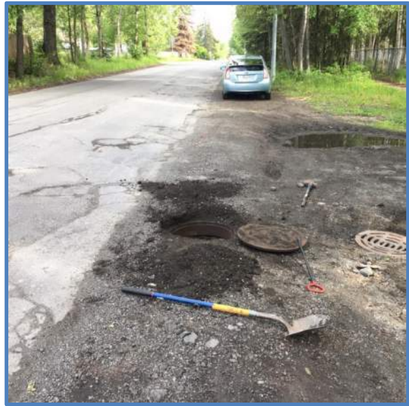
Photo 2 - Manhole / Surrounding Area
