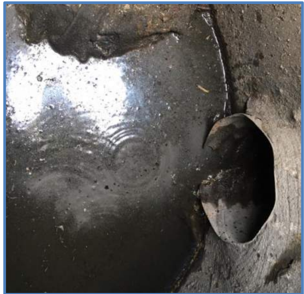
Photo 4 - Outlet Pipe Penetration
