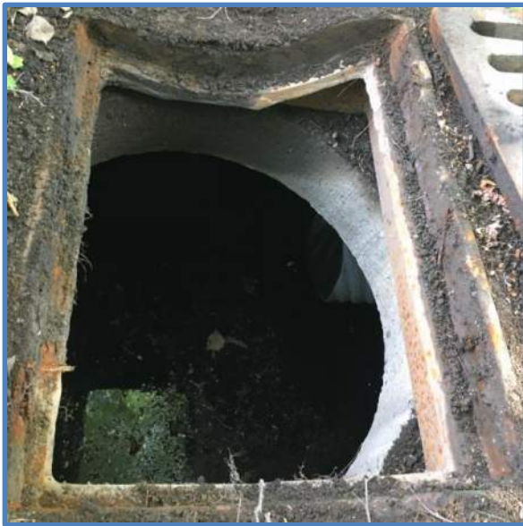
Photo 3 - Frame & Reducing Slab
