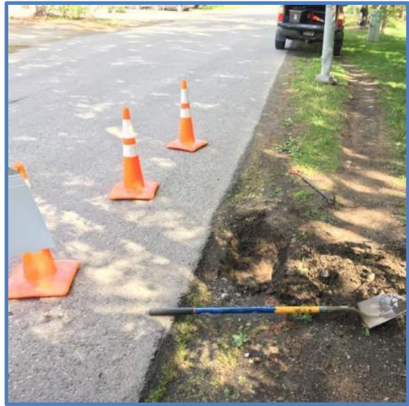
Photo 2 - Manhole / Surrounding Area
