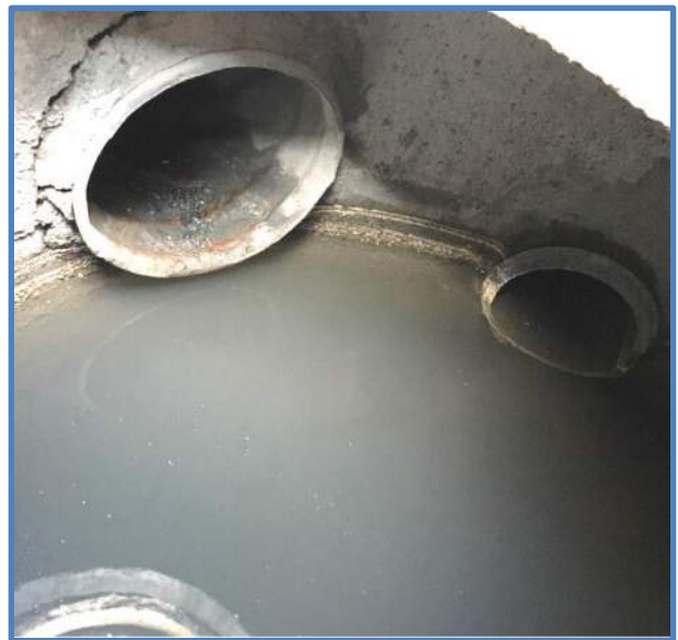
Photo 4 – West Inlet Pipe, Unidentified Northwest Inlet Pipe & Pipe Penetrations
