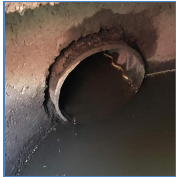
Photo 4 - Outlet Pipe Penetration
