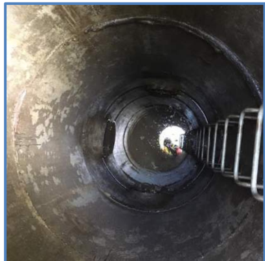
Photo 5 - Inlet & Outlet Pipe Penetrations
