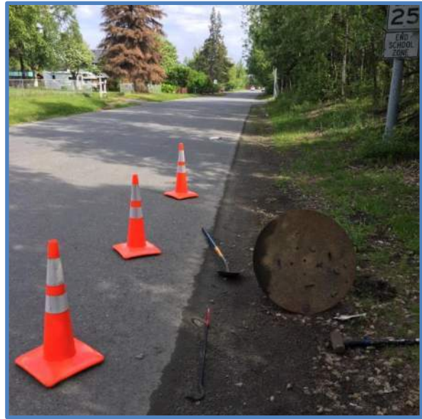
Photo 2 - Manhole Lid / Surrounding Area
