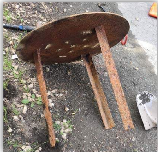
Photo 4 - Non-standard Manhole Lid
