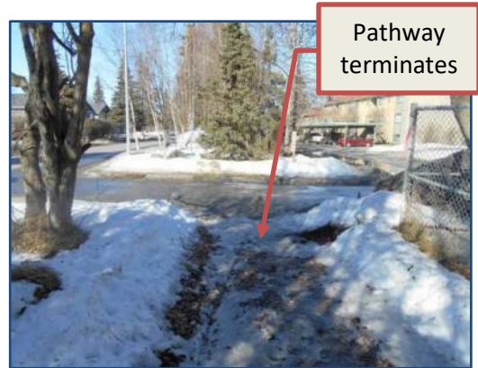
Pathway along Lois Drive is not continuous
