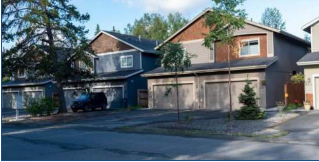
Duplex residential conditions on west side of Lois Drive
